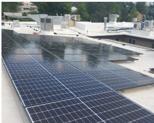
Solar Panels installed on part of the roof.
